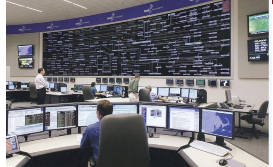
ISO New England Control Room
